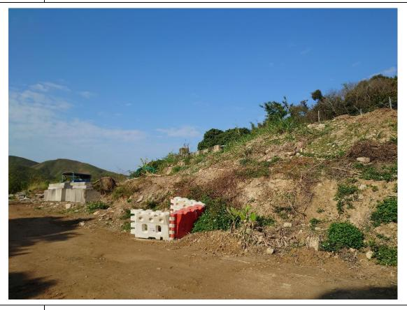
Plate 6 Front view of the partially constructed concrete block retaining wall
